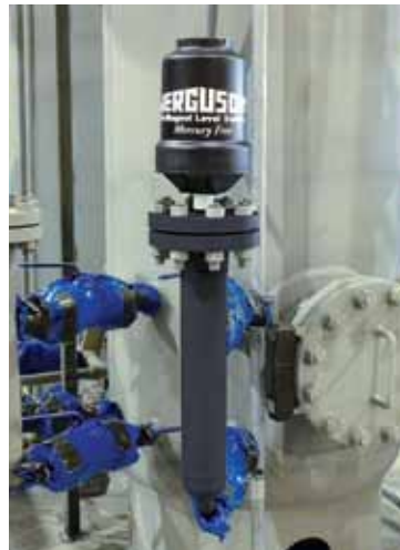
Tri-Magnet level switch and float chamber
