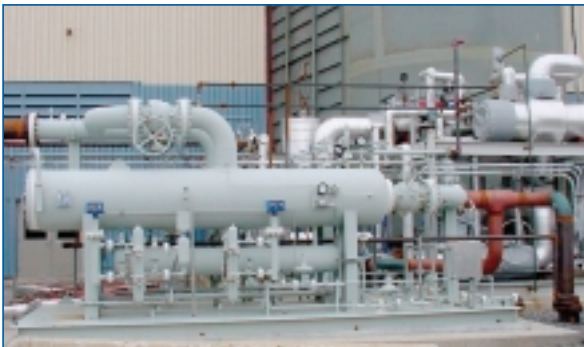
Duplexed Horizontal Filter/Separator
